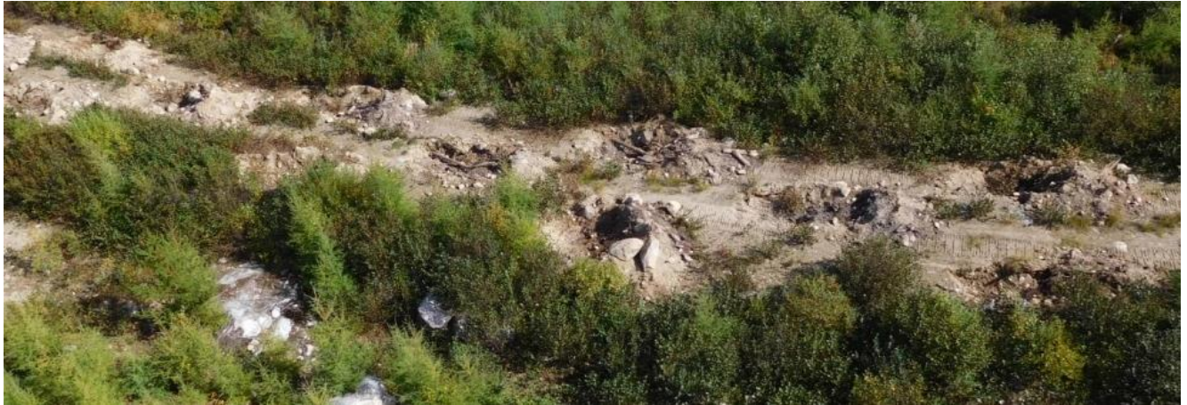
Figure 2: Road decommissioning along Spino Road
