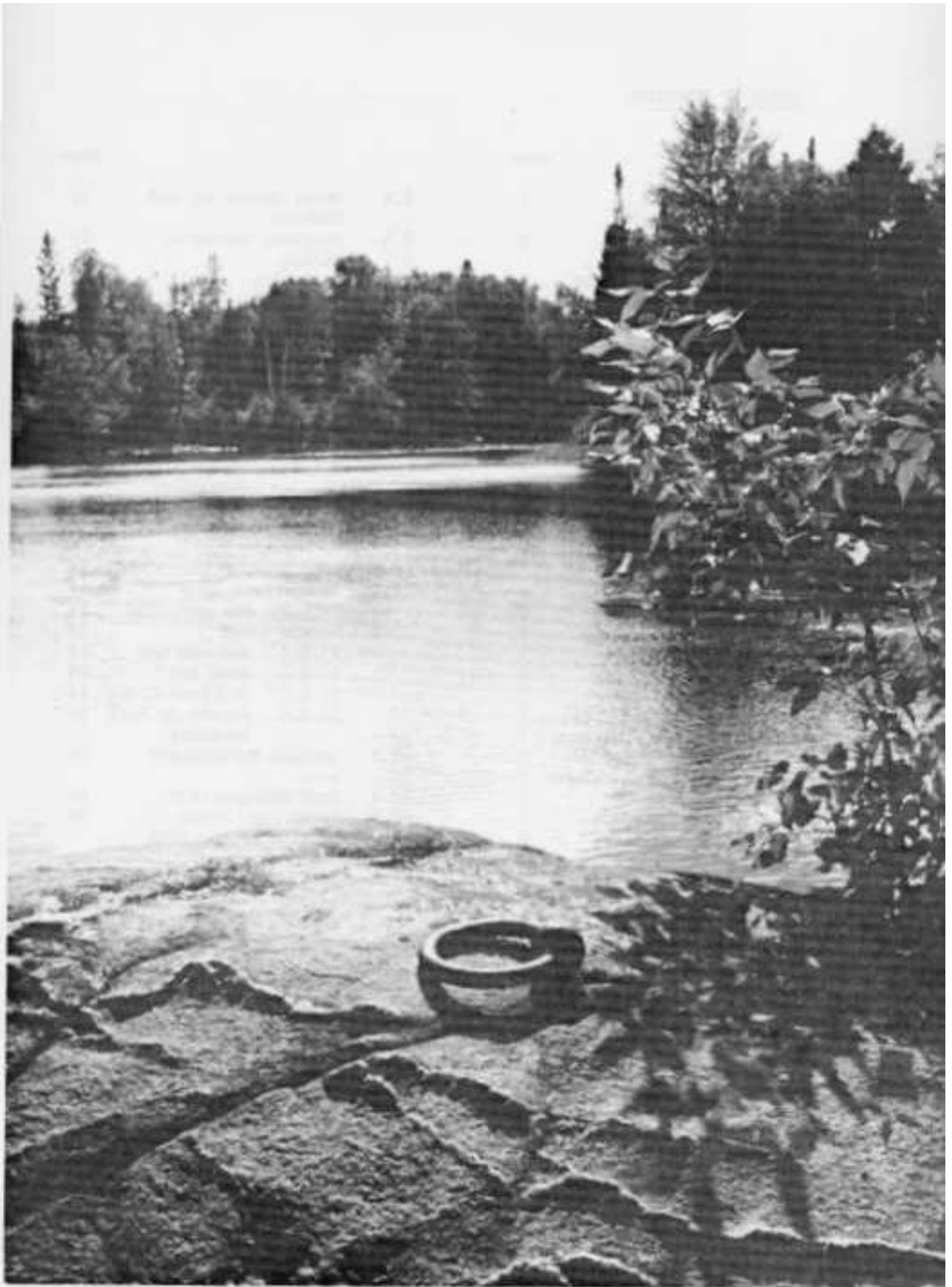
Boom ring at the head of Slate Falls
