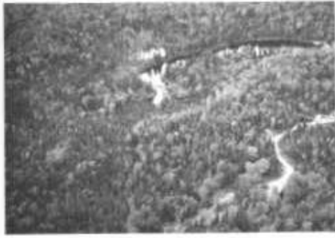
Sand River Forest Access Road
