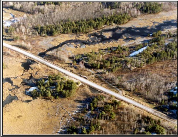
~ Located east of Highway 64 is an old MTO road bed, which provides access to Muskrat Creek ~
